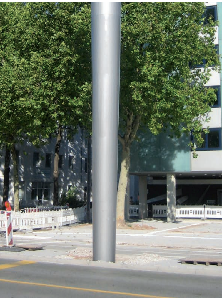
Description. Monopod Steel S235. Height 13m.
