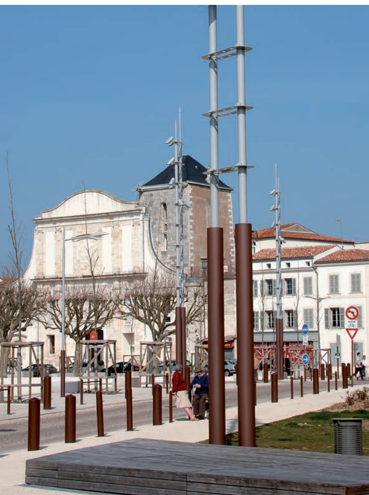
Description. Bipode Trisection S235 Steel. Plates Aluminium 6060T6. Height 14m.
