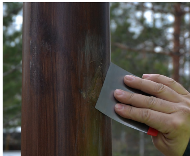
Applying epoxy
