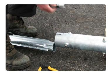
5. Tie the lifting belt onto the pole and lock the lifting hook to upper part of the hand hole
